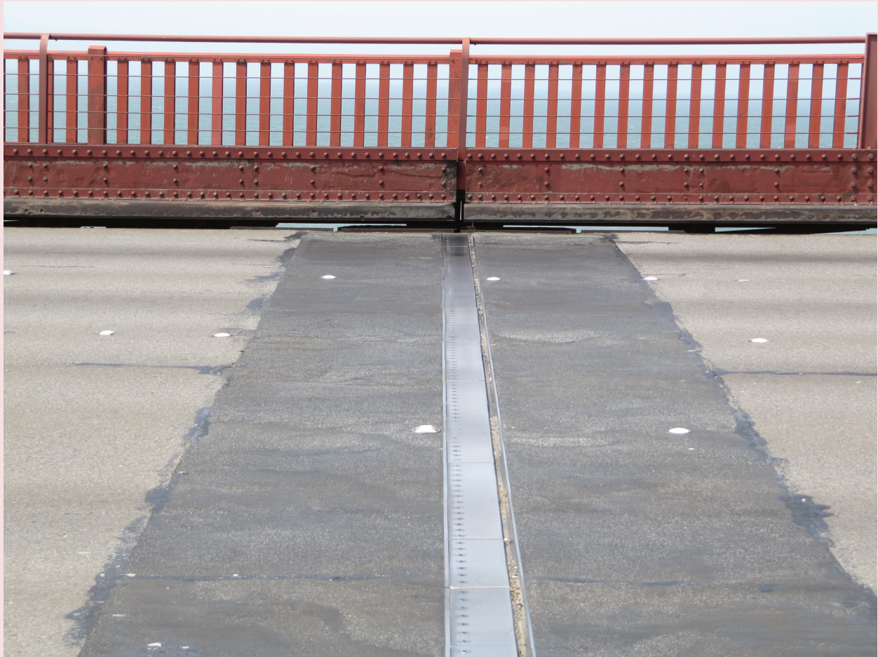
Expansion joint on the Golden Gate Bridge. Image Credit: Expansion Joint Golden Gate Bridge by Michiel1972 via Wikimedia Commons
