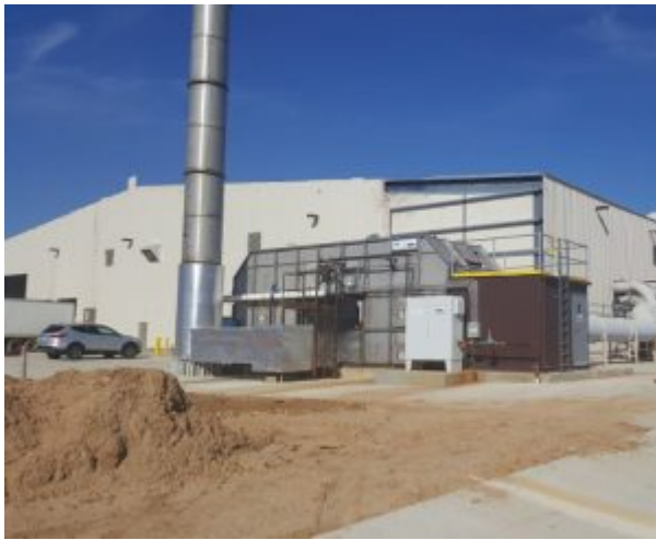
Figure 2: Air pollution control system, known as a thermal oxidizer, decomposes hazard gases from industrial air streams at a factory in the United States. By Combustion2016 – Own work, CC BY-SA 4.0, https://commons.wikimedia.org/w/index.php?curid=52028818
